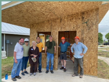
Community First Village House build
